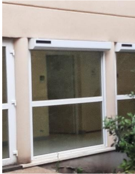
Stores service Laennec
